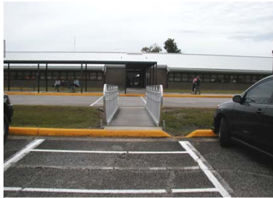
A new bridge in the parking area was not installed flush to grade
